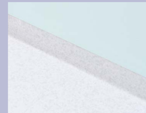
Perfect coving and hot welding
